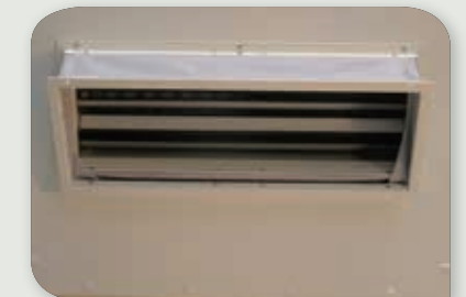
Inlet/Outlet air flange soft connection
