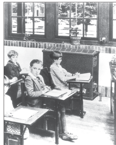
In 1917, McQuay provided the air ventilation units for classrooms.
