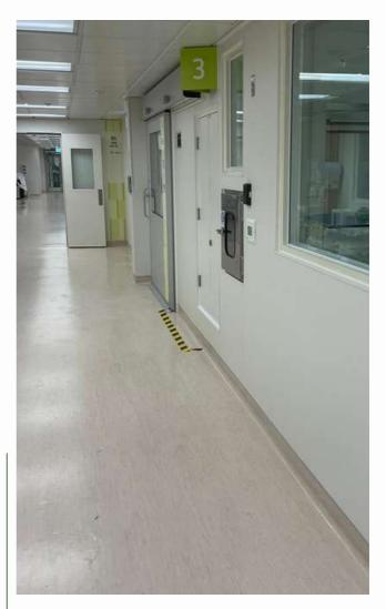
Furthermore, the lightweight feature of SPC wall panel [21kg for dimension (w)1.2m \* (h)2.4m\*(t)3.6mm), allow labour to carry out easier on site, production capacity is thereby enhanced.
